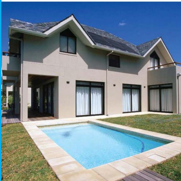
Solar Pool Collectors
